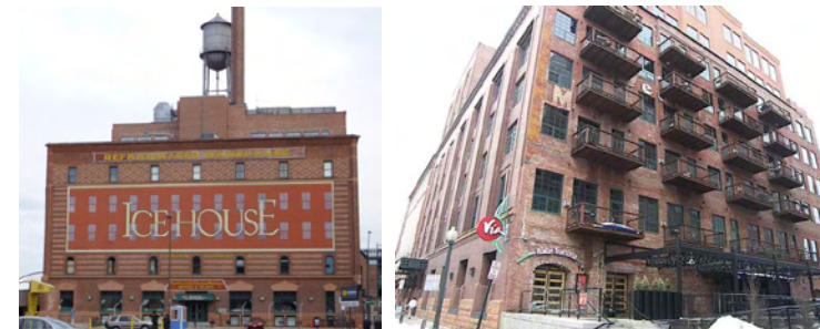
Above, the Denver Ice House and Tavern. Note the significant modification of some of the façades to accommodate housing (windows, balconies) while retaining some historical character and material references. The large super graphic "Ice House" is utilized on one of the more visible façades.
