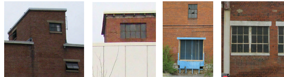
Above, images of the variety of windows and openings along the Ice House Complex historic façades. While the majority of the historic Ice House Complex façades have minimal apertures, these windows and loading docks provide plenty of formal and aesthetic references for application to the blank brick façades. Window size and placements will be a balancing act between historic references and allowing natural light for people living and working within the Ice House Complex.
