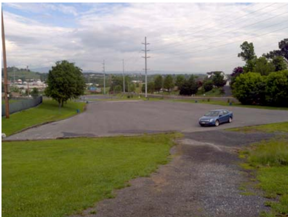
Existing softball field parking and access
